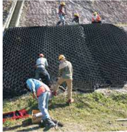
Process of hydroseeding
